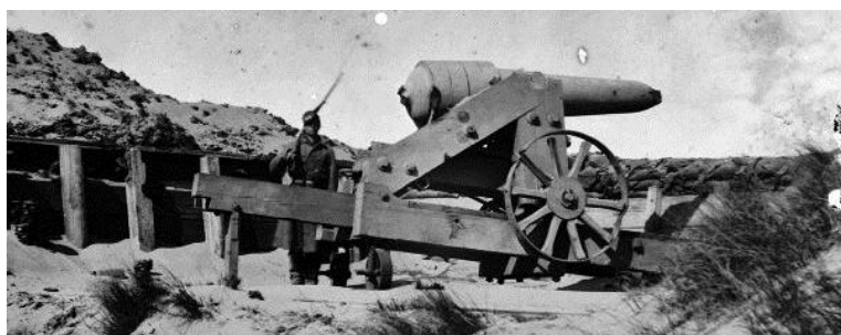
Fig. 62. Fort Fisher Muzzle damage
